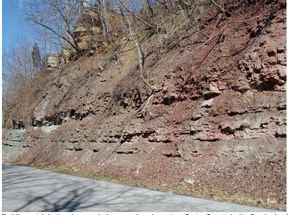
Red (iron staining) and green shales, seen here in eastern Carter County in the Cumberland Plateau Region, are low strength, sensitive to moisture, and prone to slumping and land-slides. Photo by Jerry Weisenfluh, Kentucky Geological Survey.
